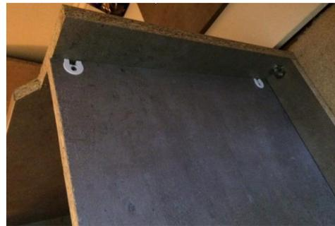
8. Carefully stand unit upright (suggest two people), place in position and fix to wall using L brackets or aluminium channel if supplied.
