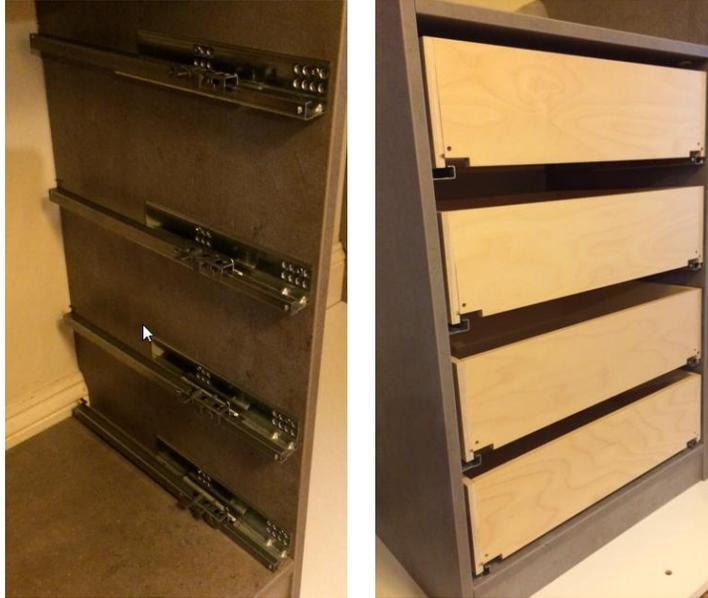
12. When the box is sitting nice and square push the rod at the front of the runner into the pre drilled hole in the bottom of the box (on both sides).
